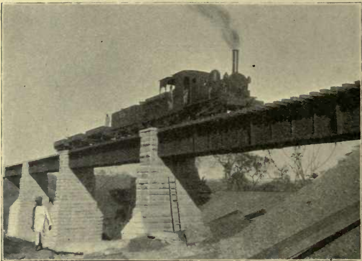
"VERY SOON I HAD THE SATISFACTION OF SEEING THE FIRST TRAIN CROSS THE FINISHED WORK."
