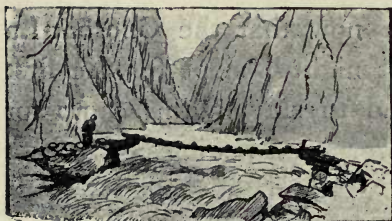
“AT LAST A NEW BRIDGE WAS COMPLETED.”
