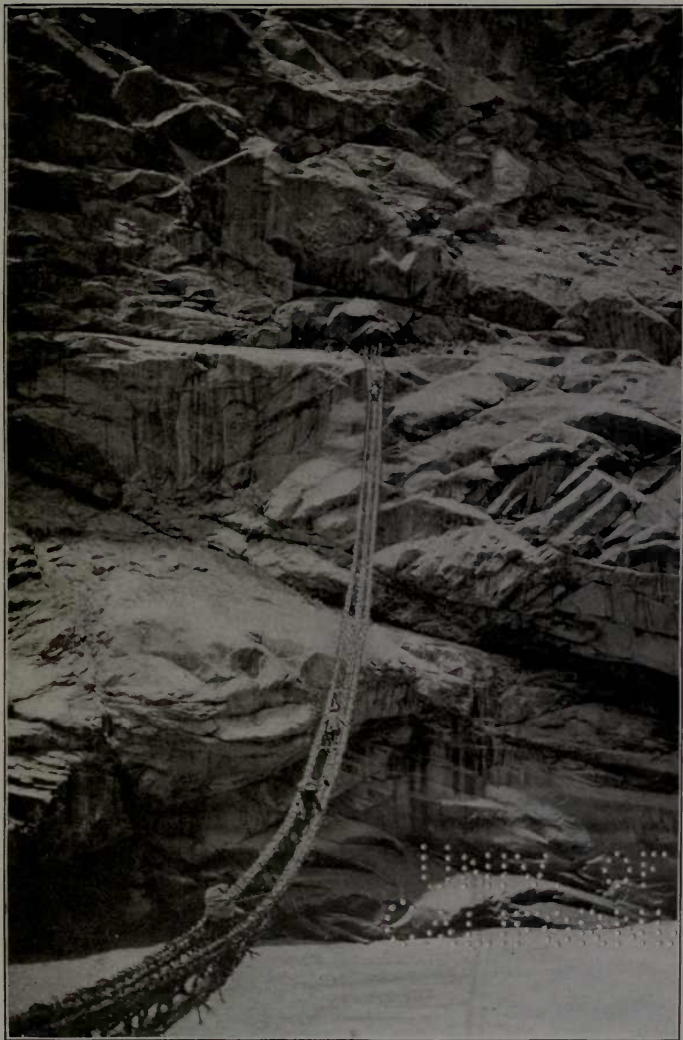
TAKEN FROM THE CENTRE OF THE ROPE BRIDGE
