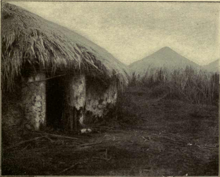
TYPICAL NEGRO HUTS MADE OF UPRIGHT STICKS PLASTERED WITH MUD AND THATCHED WITH REEDS
