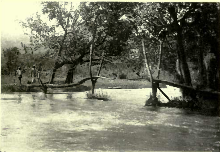
THE CENTRE OF THIS BRIDGE WAS WITHDRAWN AT NIGHT SO AS TO KEEP MEN AND BEASTS FROM CROSSING OVER TO THE ISLAND
